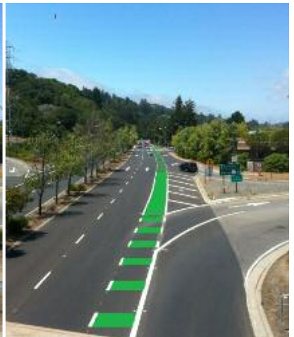
The proposed green striping along the bike lane on Camino Pablo, and proposed location change, pictured, are scheduled to be discussed at the Aug. 18 Orinda City Council meeting.
